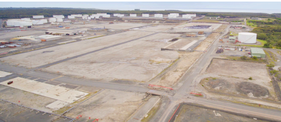
BESS investigation area within the Ampol Kurnell Terminal
